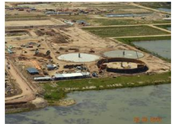
Water and effluent treatment plant
